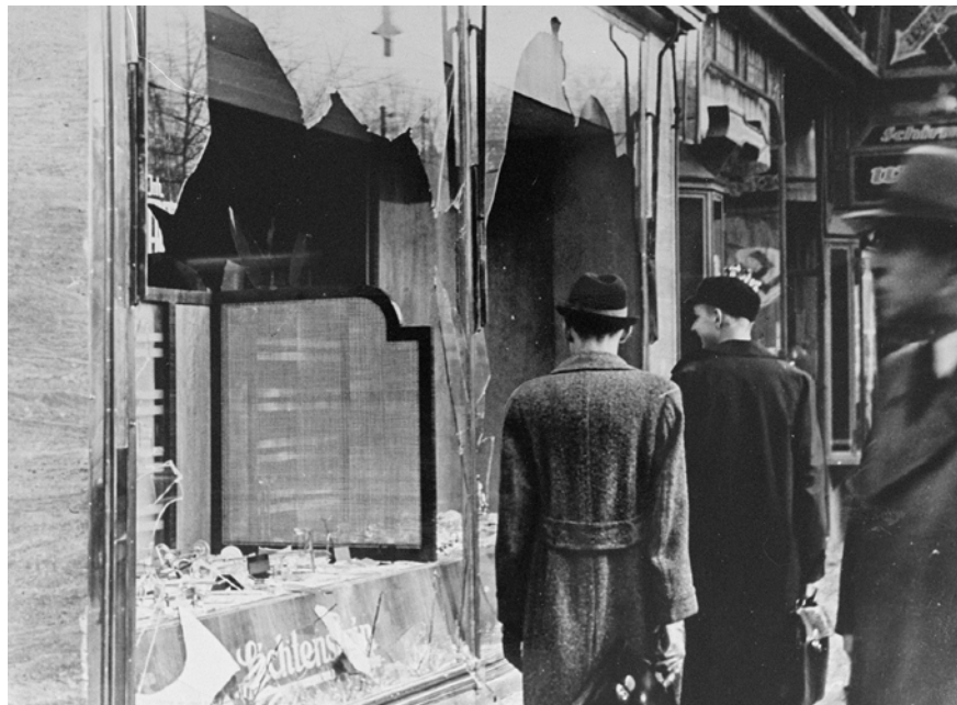
Germans pass by the broken shop window of a Jewish-owned business that was destroyed during Kristallnacht. Photo Source: National Archives and Records Administration, College Park
