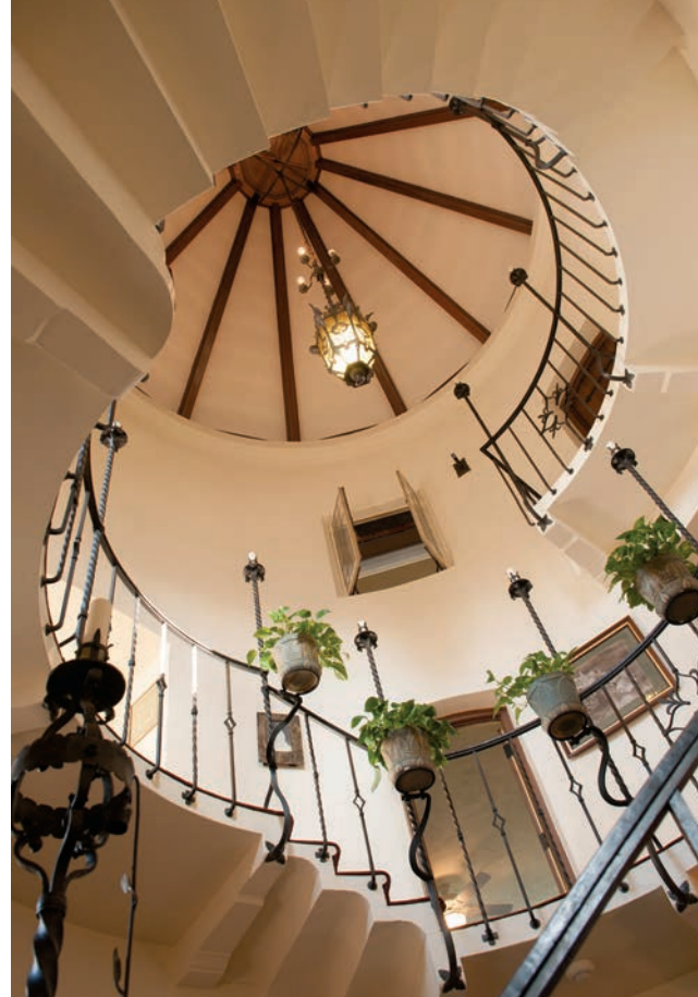
The spiral stairway, right, rises up three floors. The wrought iron railings and candle fixtures were custom-made for the home. The stairs are concrete.
